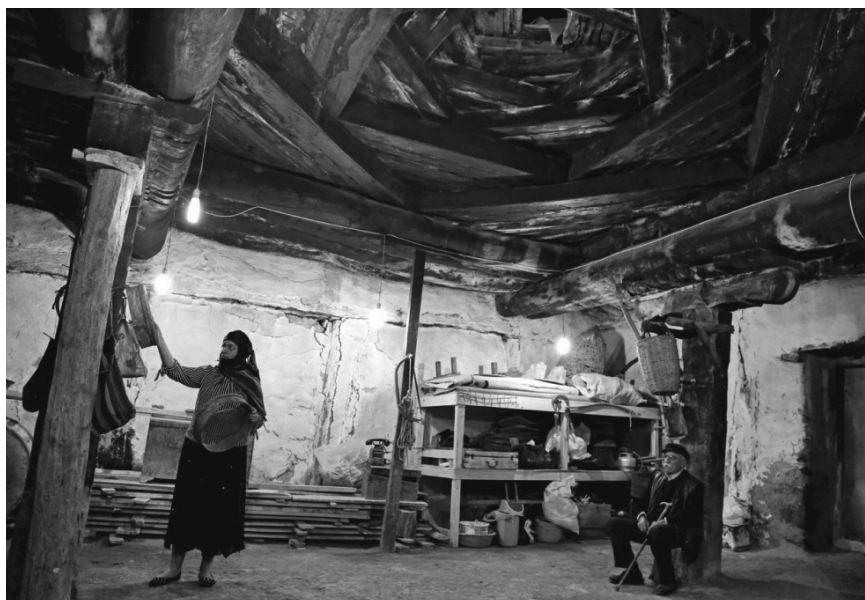
Figure 6.1 A building with a multi-layer roof signifying the seven heavens ( kırlangıç çatı ) used for cem gatherings in the past, Zara-Sivas
